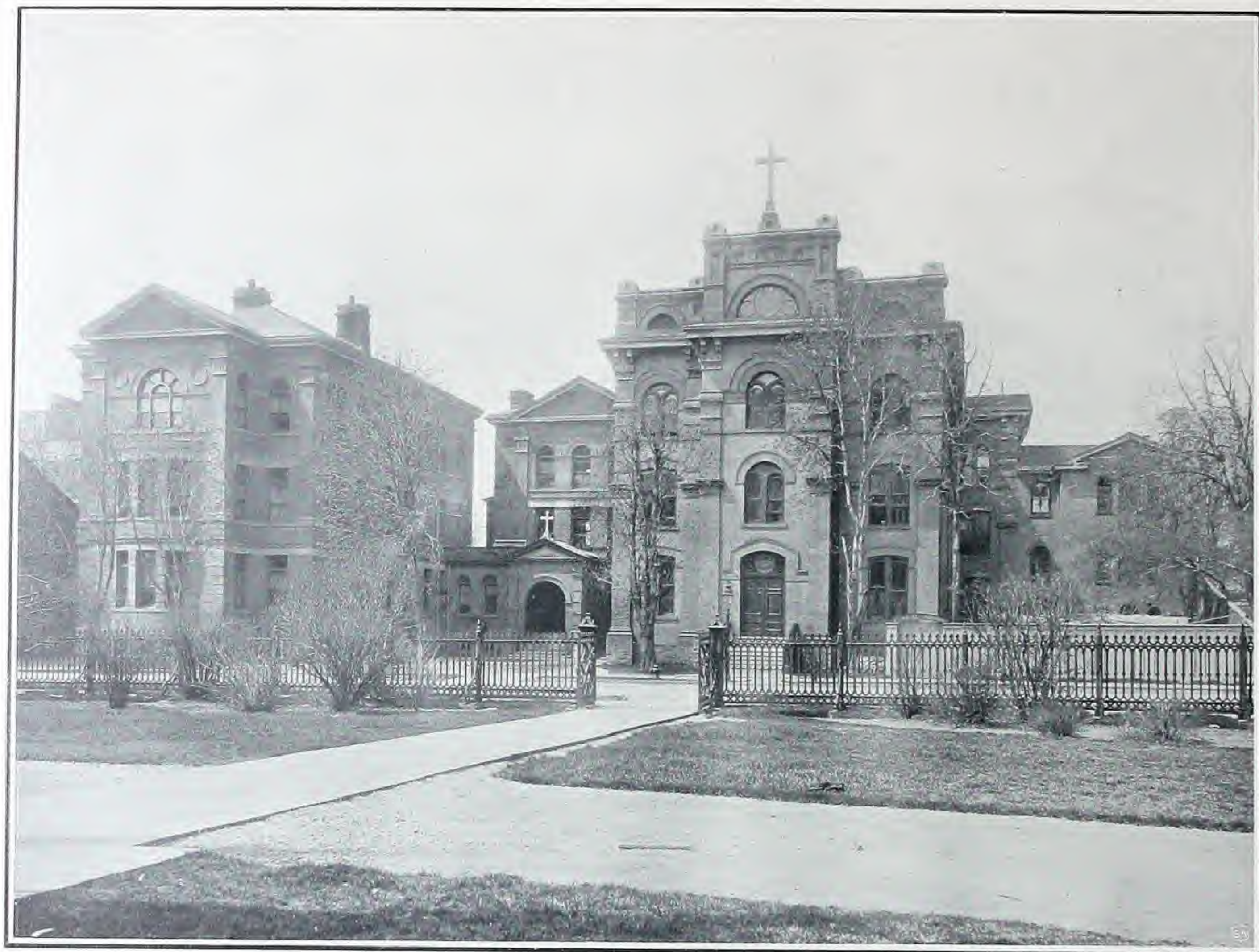
Fig. 182. —St. Michael's Hospital, Toronto In which the "Hayes" Patent Lathing was used.
